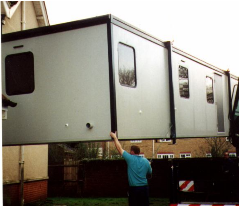
The Portacabin being off- loaded
